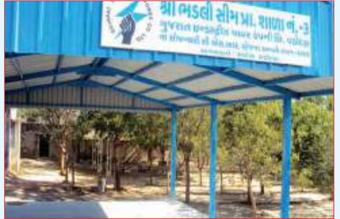
Construction of School Shed, Bhadli
