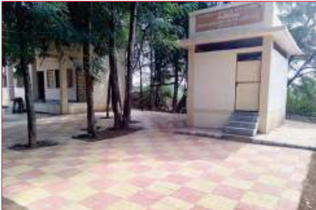
Providing and laying Paver Block, Nani Naroli
