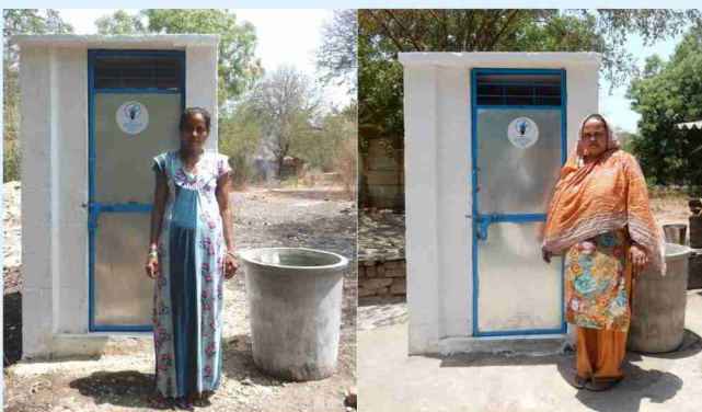
Construction of Toilets - Village Dungri, Taluka Mangrol, District Surat
