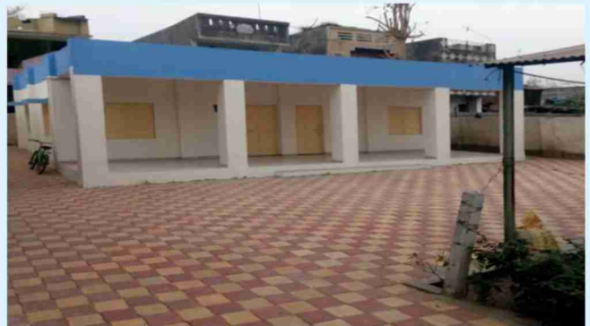
Construction of Class Rooms, Primary School, Village Dhanora, District Vadodara
