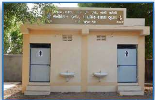
Construction of Sanitation Unit, Primary School at Village Luna, Taluka Valia, District Bharuch
