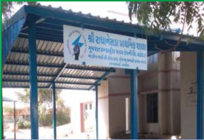
Construction of Shed Shree Raghnesda Primary School
