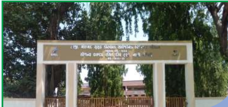
Construction of Main Entry Gate, Baudhan High School
