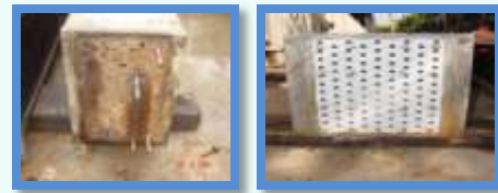
Cooler Before & after Cleaning
